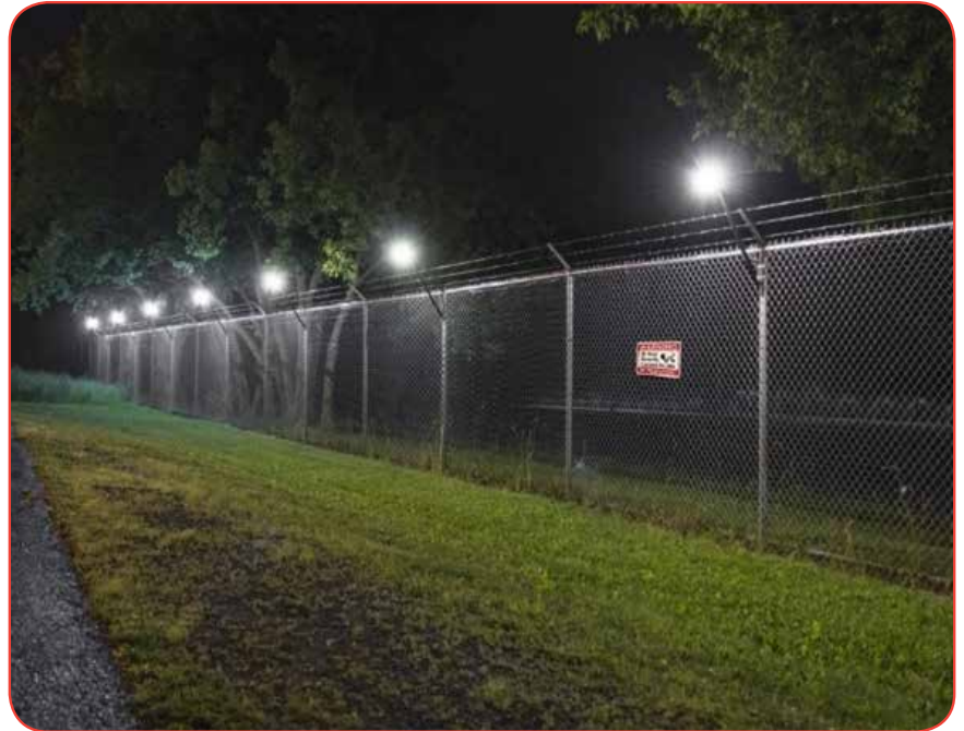
Intelligent lighting system illuminates the fence line, detects intrusion attempts, and deters intruders by strobing or increasing intensity at the intrusion location
