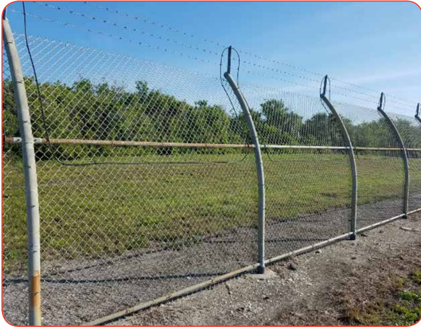
A high-security fence enhanced with a fiber optic perimeter intrusion detection sensor. Any attempt to cut, climb, or lift the fence fabric is immediately detected
